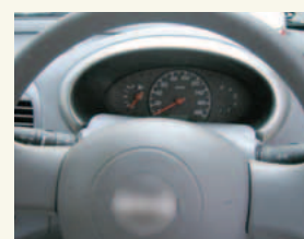
Fixing sound absorption materials around instrument panels
